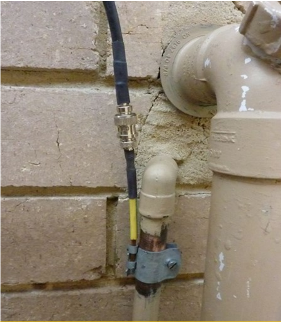
Water pipe termination.
